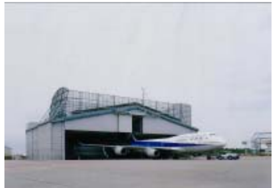
Hangar type noise suppression facility (Narita)
