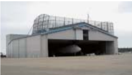
Noise reduction hangar at Narita Airport
