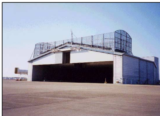
Hanger type noise suppression facility (Narita)
