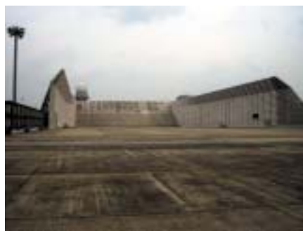
Engine test facility with soundproof walls at Osaka Airport
