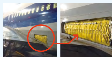
Boeing 767 With Missing Panel
